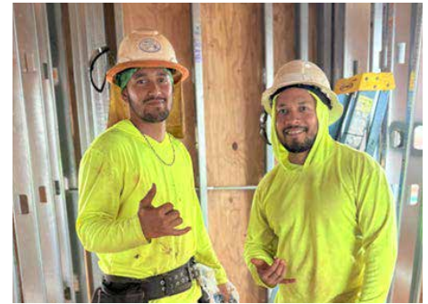
Koa Ridge Walea 2. TNH Plumbing. GC: Castle & Cooke. (l-r) Daryl Keawe, Forrest Gomes.
