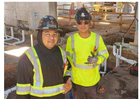
Plumbers and Fitters Local 675 New Training Facility. Alakai Mechanical. GC: Unlimited Construction. (l-r) Anthony Edrado and Zachary Clemente.
