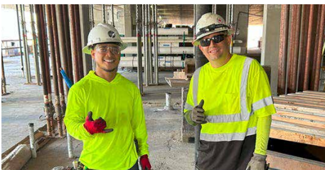
HPHA School Street Redevelopment Phase 1A. Pan Pacific Mechanical. GC: Hawaiian Dredging. (l-r) Kingsley Albano, Vince Young.
