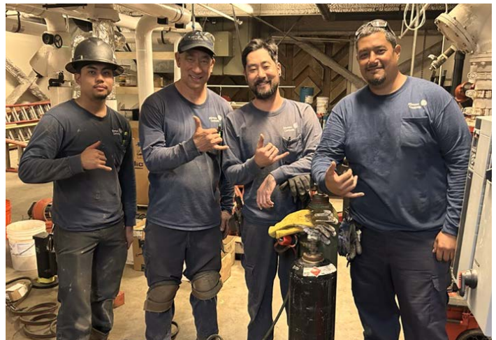
Hawaii Convention Center Chiller Replacement. Johnson Controls. (l-r) Cole Pagampao, Scott Chun, Gavin Uyeda, Kawika Johnson.
