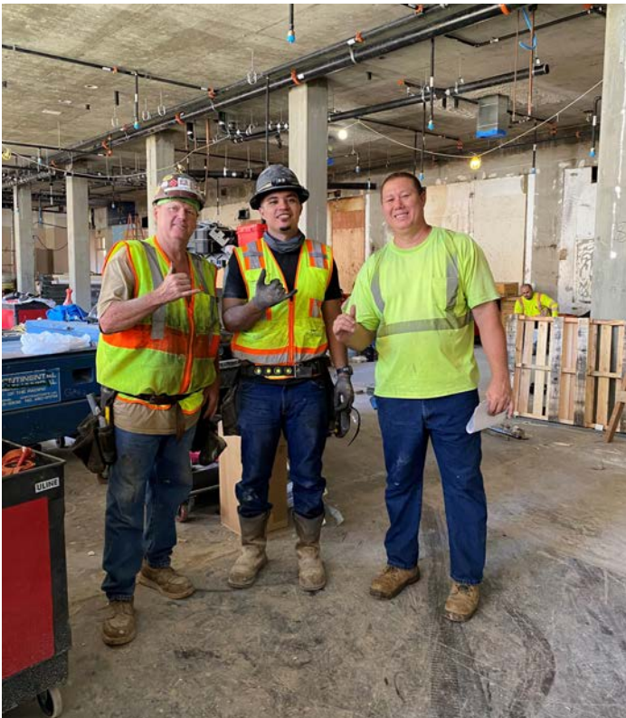
(l-r) Todd Shelton, Donovan Rogers, and Isaac Holbron. Continental Mechanical-Mechanical Fire Crew. A/C Marriott.
