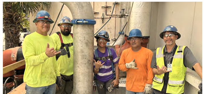
Queens Emergency Room Renovations. Dorvin D. Leis. GC: Hawaiian Dredging. (l-r) Keawekulua Leong, Micah Kahooahanohano, Makana Angay, Jason Kim & Randy Yamauchi.
