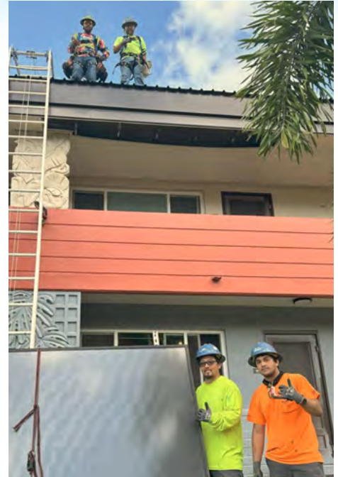
Palolo Valley Homes Renovation. Dorvin D. Leis. GC: Arita Poulson. (Roof top l-r): Turaihere Galzote, Darren Kawamoto. (Ground level l-r): Chad Yamashita, Chastin Baquiran.
