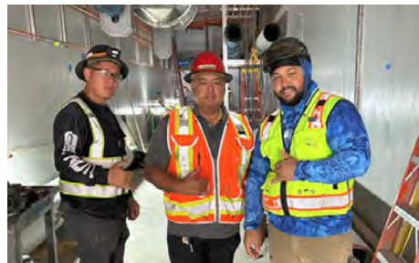
Sand Island Wastewater Treatment Plant - Phase 1. Pan Pacific Mechanical. GC: Hensel Phelps.
