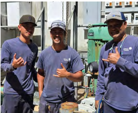
Hapuna Condenser Water Pump Overhaul in Kona. Johnson Controls. (l-r) Boston Matsu, Byron "BJ" Freitas, Keith Bermudez.
