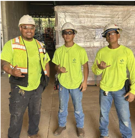
Halawa View Apartments. Commercial Plumbing. (l-r) Sosia Havea, Shaun Lee Saito, Clarence Bareng. GC: Nordic PCL.
