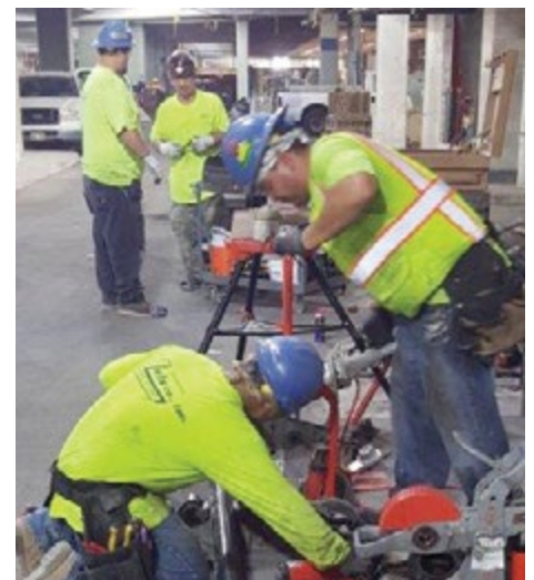
Dorvin Leis' workers busy at work.
