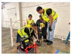
Alan Ibanes (instructor) – Students using the drain camera/toner to locate the piping under the flooring, then using blue tape to layout the piping.
