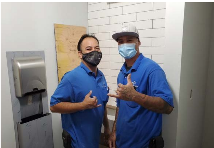
(l-r) Troy Lum, Warren Ballesteros. Commercial Plbg. Hemic Building Renovation. GC: Kadowaki.
