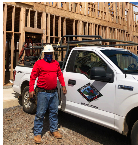
Layton Aguon. Diamond Plumbing Co. Koloa Village. GC: Shioi Construction.
