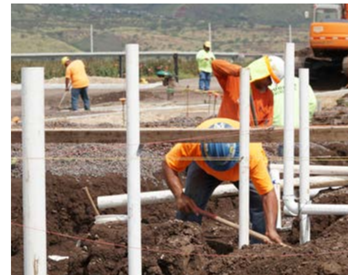
Crews from TNH Plumbing preparing the foundation for more housing units.
