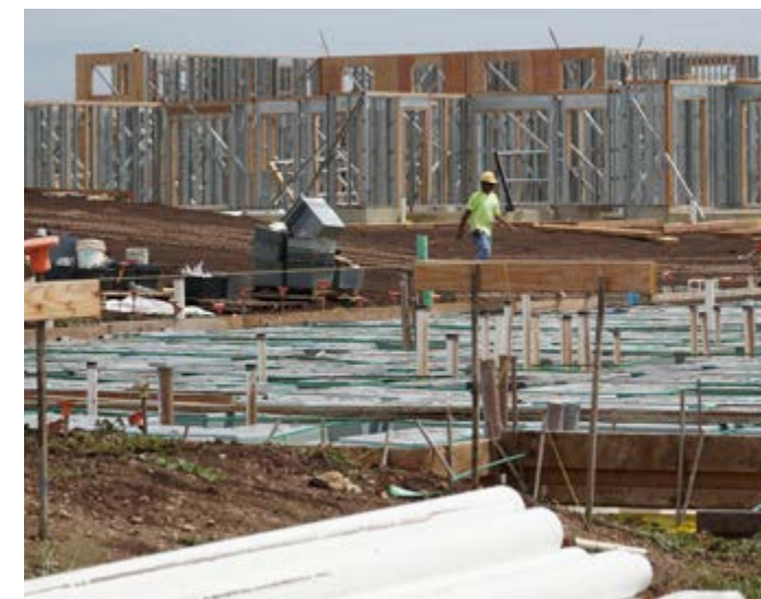
Industry trades working on different areas of Ho'opili.
