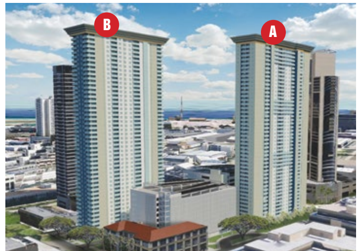
Work on Tower B for the 801 South Street condo complex was held by a court order based on complaints state law was not adhered to. A review is pending and work resumption is expected.
